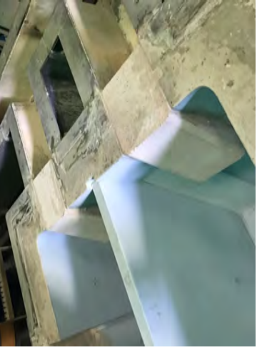
Installed airlocks and closed bolt holes with duct-tape
