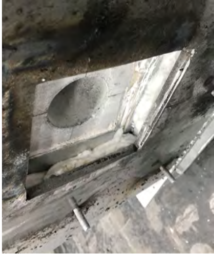
Stuffed active gravity drain port and gravity drain spacer installation
