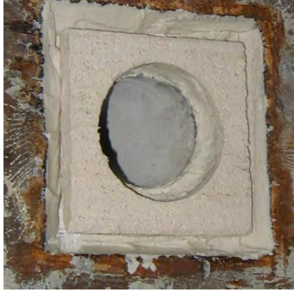
Gravity drain spacer installation
