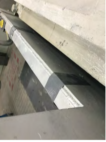
Installed airlocks and closed bolt holes with duct-tape
