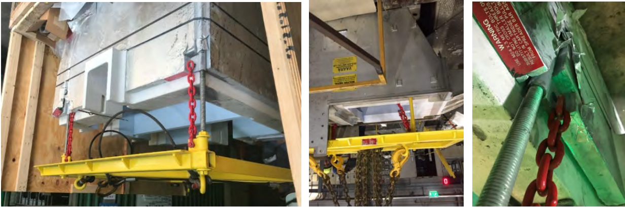
Spreader bar installation
