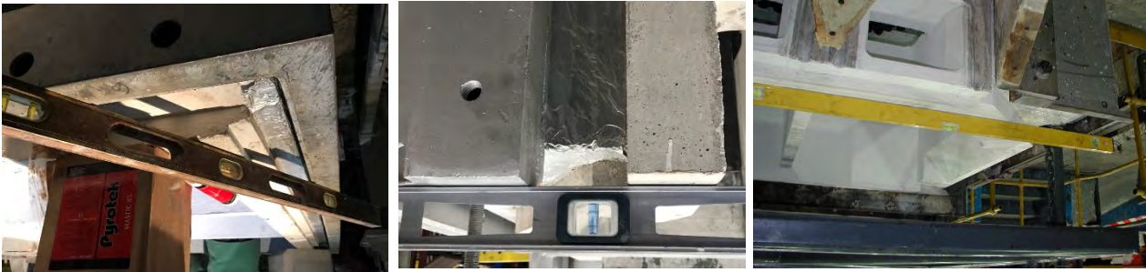
Leveling the new cartridge and steel shell
