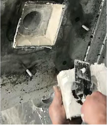
Stuffed active gravity drain port and gravity drain spacer installation
